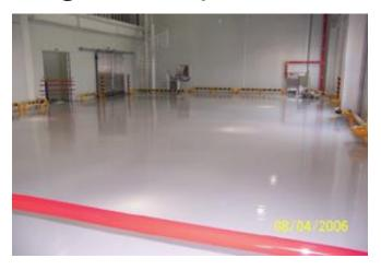
RUST GRIP ® / MOIST METAL GRIP ® application was found to excel in the adhesion to the concrete surface as well as in the toughness to pressure and abrasion when compared to the existing epoxy coating.
