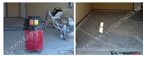
Two coats of NON-SKID ® were applied to provide durability and long lasting protection
