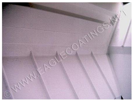
Protected with a top coat of RUST GRIP (6,750 psi ) @ 5 - 8 mils WFT = 2 - 4 mils DFT or 200 sq. ft. per gal.
