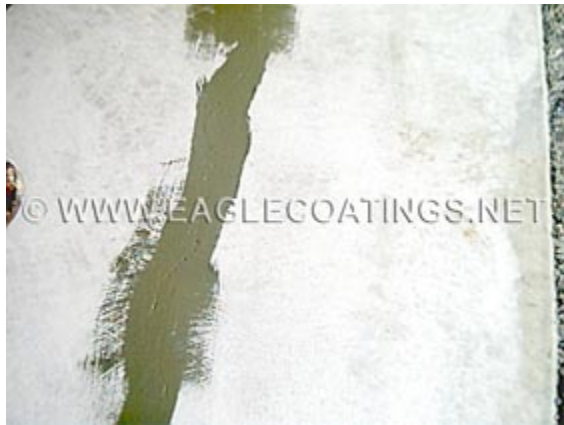
Patch and Pre stripe the cracks
