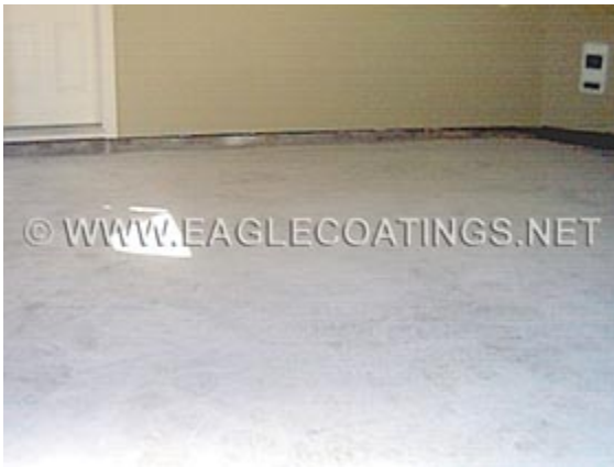
Prepare surface with grinder
