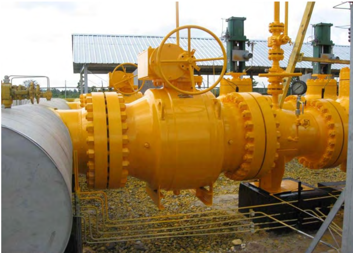
Application of Enamo Grip (safety yellow)
