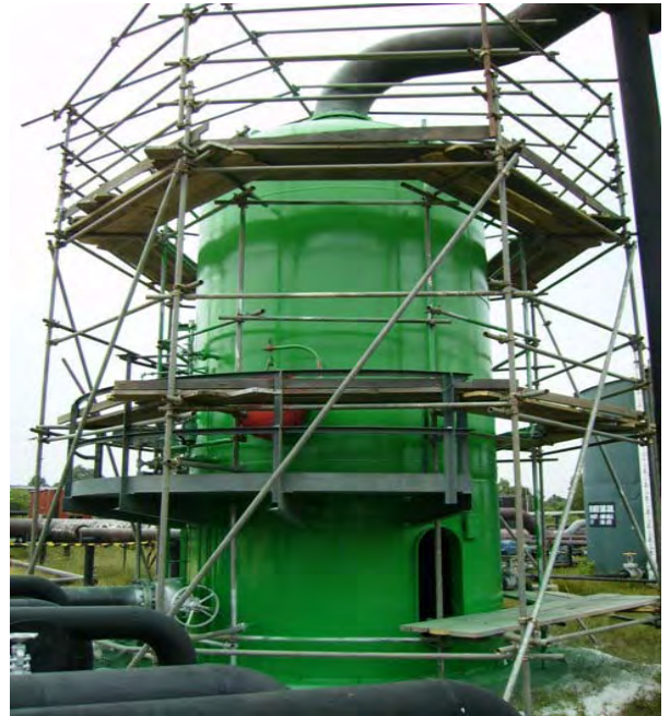
Completed Project - Rust Grip® and Enamo Grip
