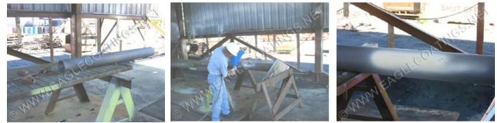
Temperature reduced from 350°C on the bare pipe to 170°C after the initial primer coat @ 50 mils/1.27 mm DFT.
