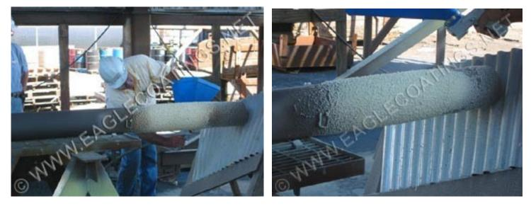
A temperature reduction from **395°C** on the bare pipe to **55°C** after the build coat @ 100 mils DFT was applied.
