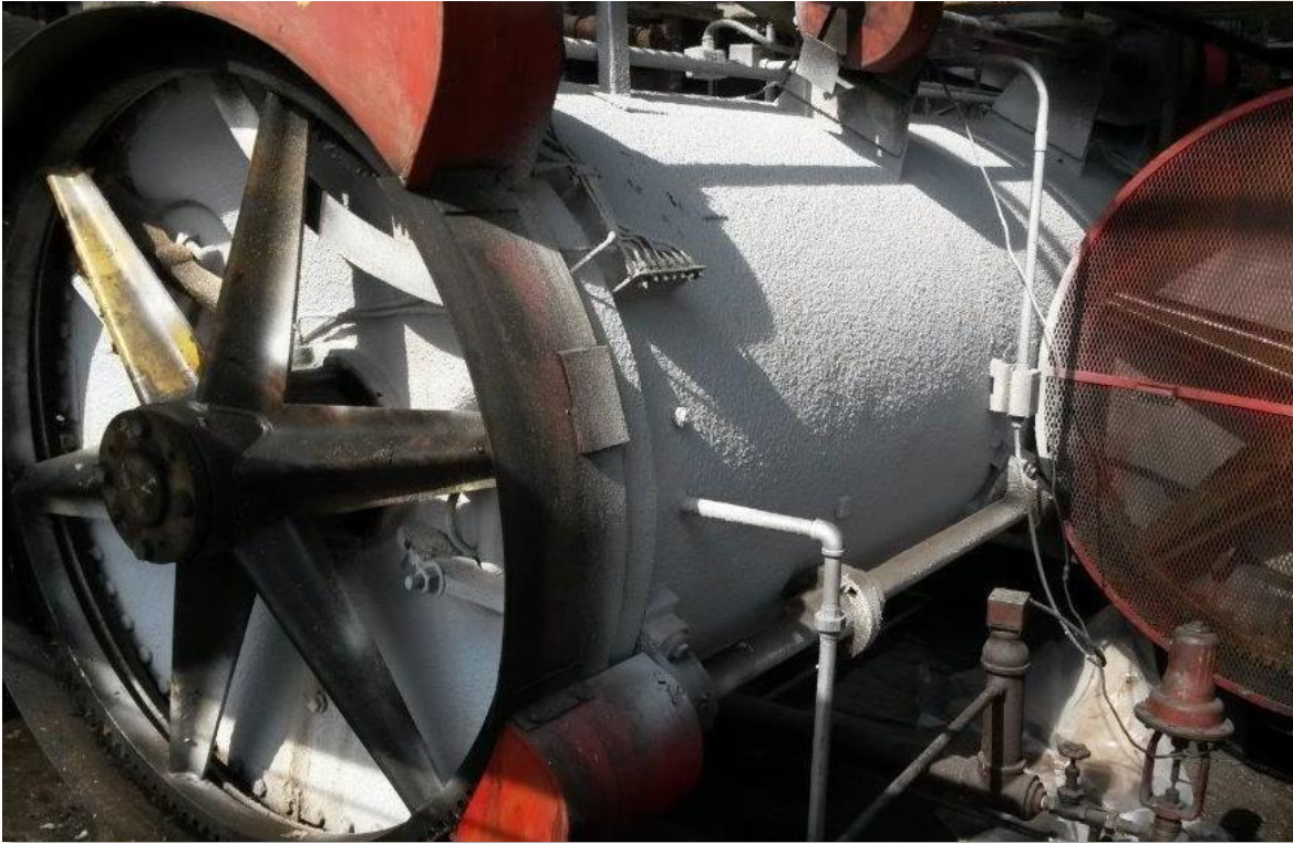
Close-up of application HOT PIPE COATING
