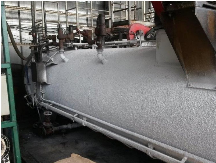
After application HOT PIPE COATING
