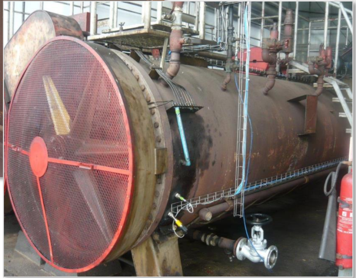
Installation prior to application
