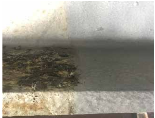
Right Side of Beam
