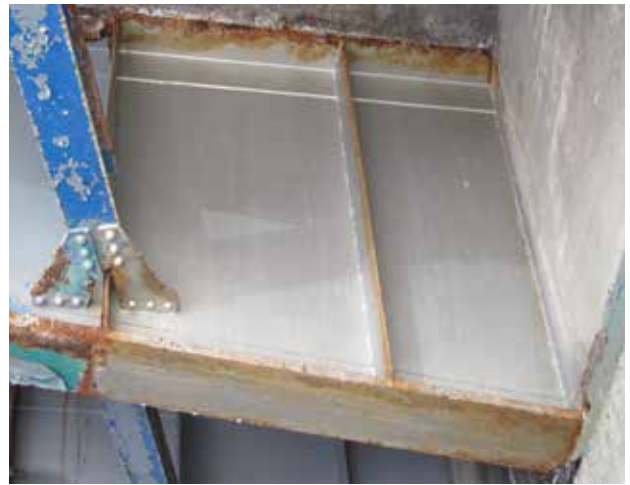
Rust Grip ® Application 09-14-17
