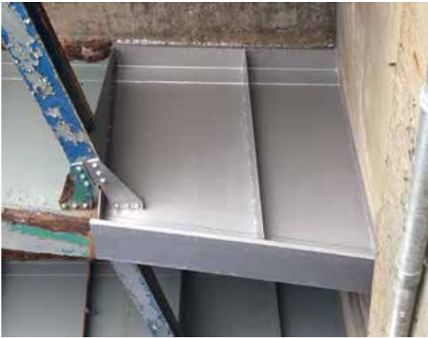
Rust Grip ® Application 09-16-15
