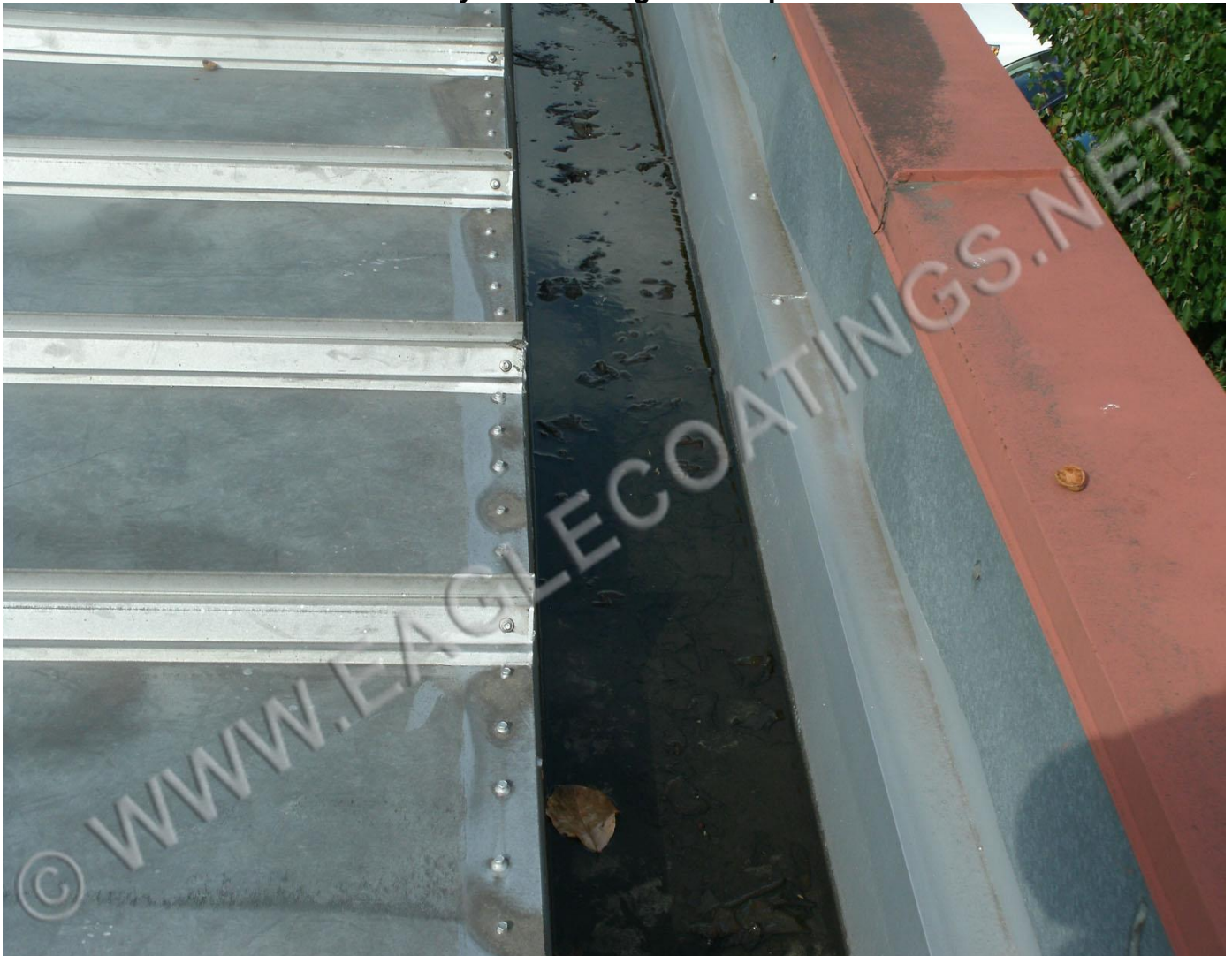
3 years of sludge build-up
