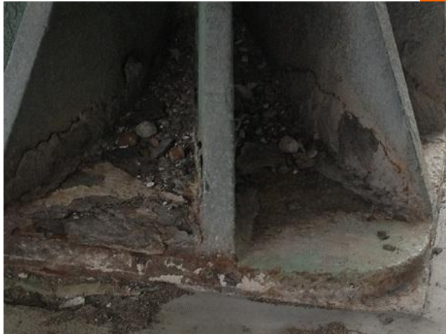
CLOSE-UP PRIOR TO RUST GRIP ® APPLICATION
