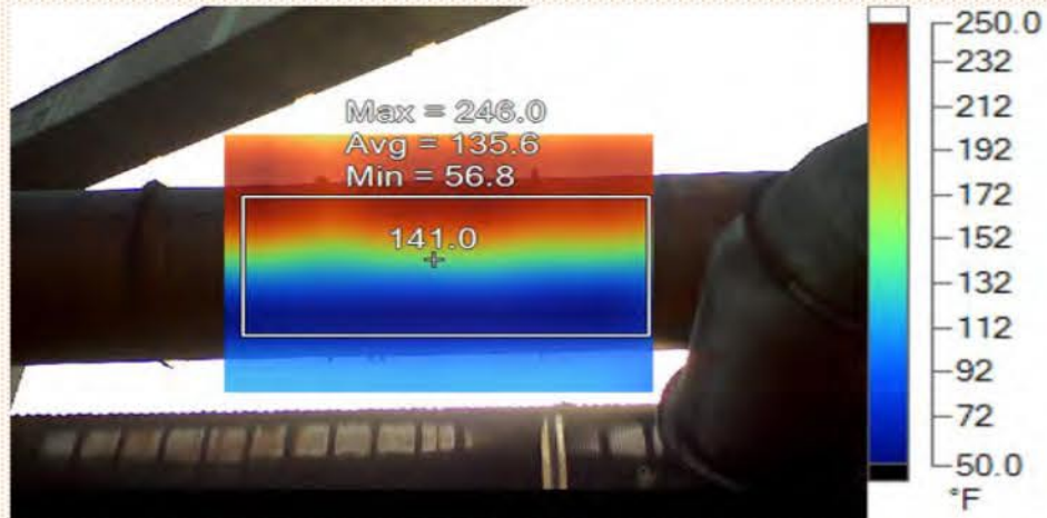
Before Ceramic Thermal Barrier Coating
