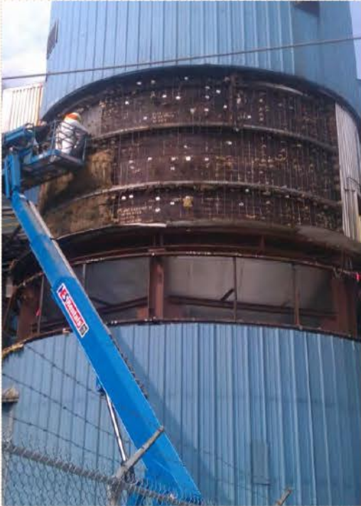
Before Traditional Mineral Wool & Cladding
