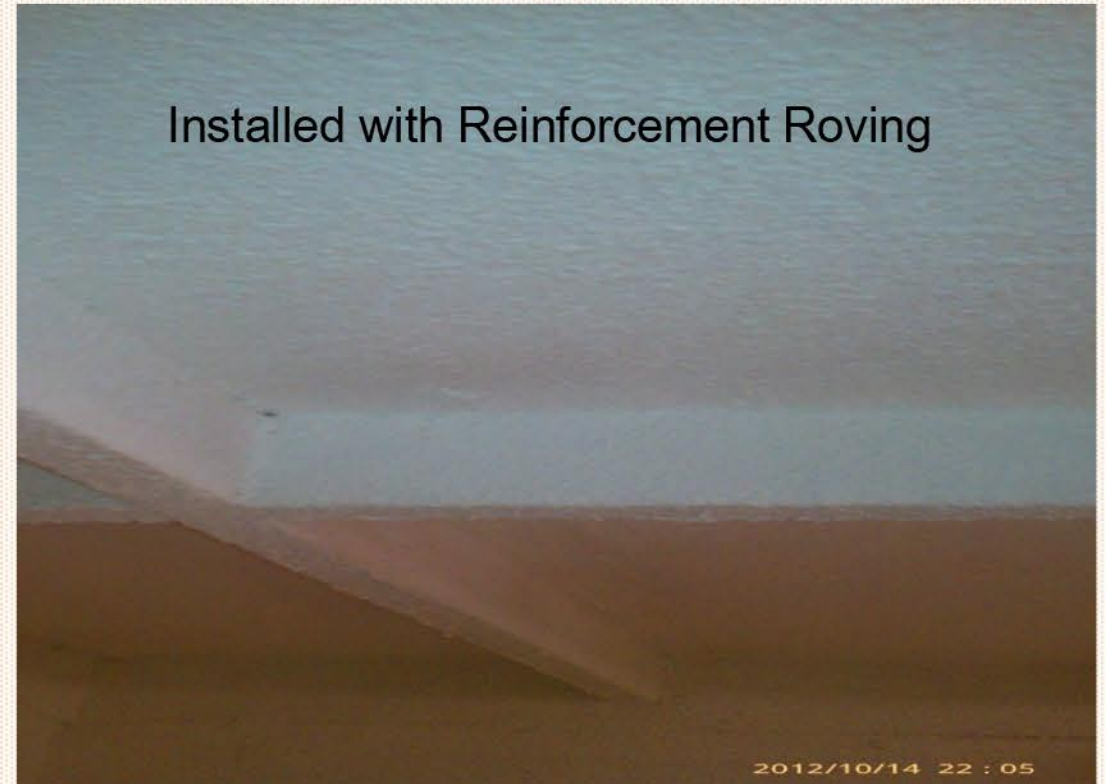
CTB-1 HS (Rust Grip – HPC- Rust Grip - Lining Kote)
