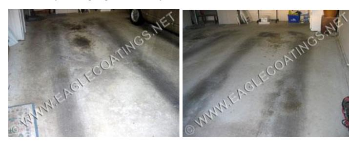
A biodegradable emulsifier was applied to the concrete surface, followed by a high pressure steam cleaning to provide a clean substrate for the application of NON-SKID ®
