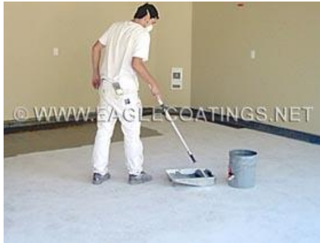
First Coat of NON-SKID®
