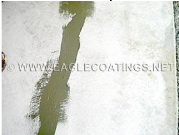
Patch and Pre stripe the cracks
