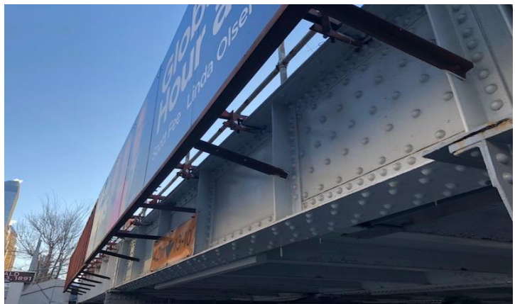
Project Details: City of Calgary - CP Rail Steel Bridge / Overpass Encapsulation of lead-based paint and rust.
