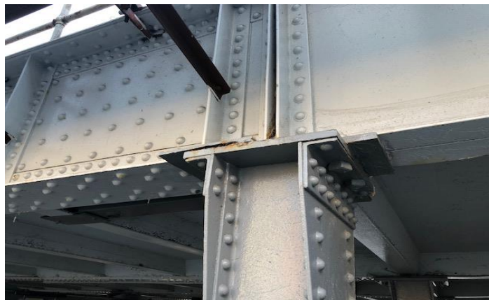
Project Details: City of Calgary - CP Rail Steel Bridge / Overpass Encapsulation of lead-based paint and rust.
