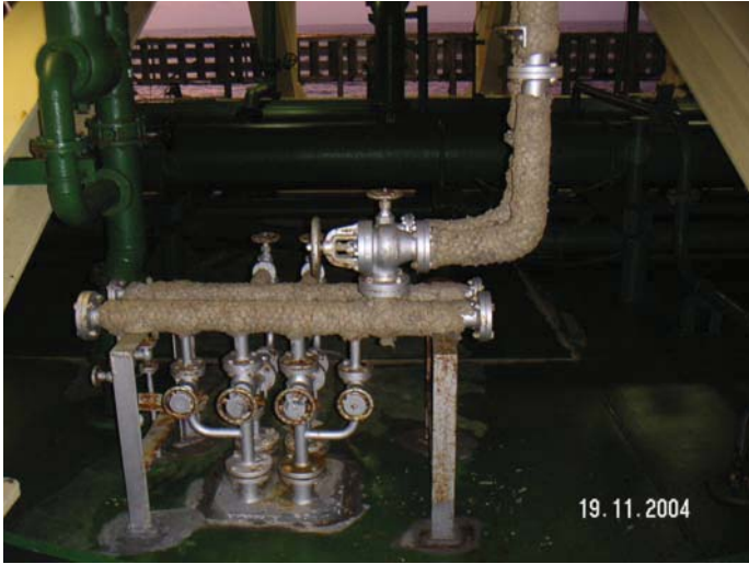
Africa – Heat Pipes Old Insulation
