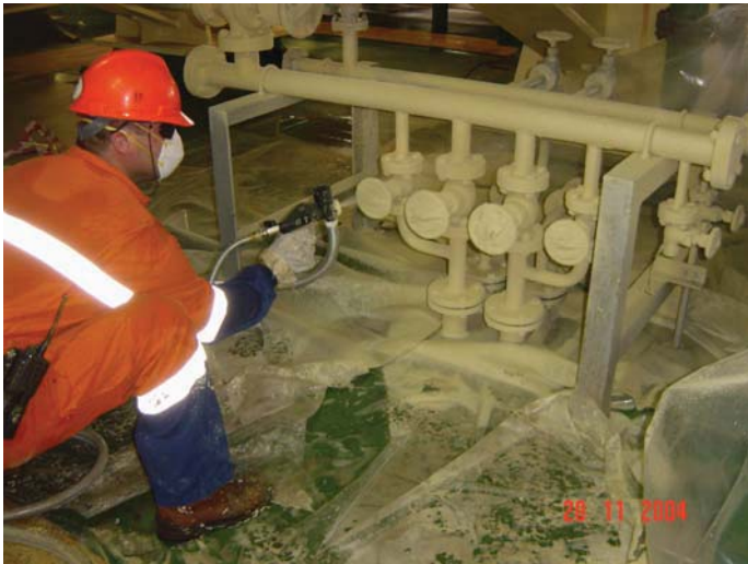
Africa – Heat Pipes After Coating Hot Pipe Coating
