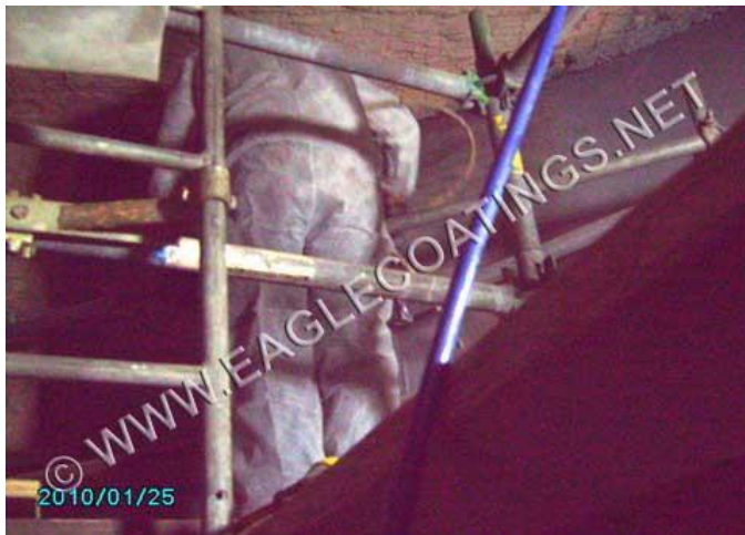
Sand Blasted Metal Surface to approximately a 2 mil profile
