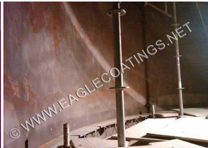
Sand Blasted Metal Surface to approximately a 2 mil profile
