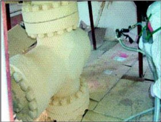
A wellhead consisting of 300mm pipes and a valve is 220C hot. The surface, which is ca. 7m<sup>2</sup>, heats up the environment and the walls of a shed, which is dome of steel and fiberglass. The heat causes damage to the fiberglass and makes work within the shed uncomfortable. The high heat also causes threat of injuries to the workers.
